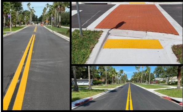
Phase 1 of the Indian Rocks Road project REOPENS 1,268 engagements
