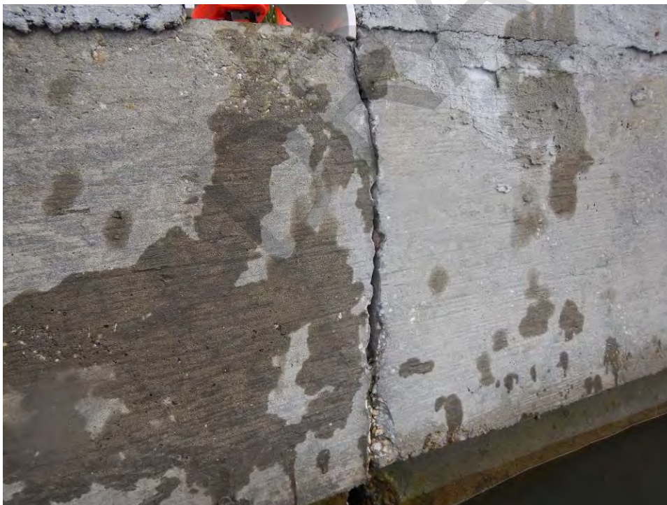
Figure 5-3: Crack in concrete panel cap at wall joint
