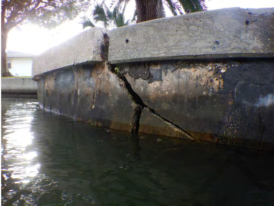
Figure 4-4: Southwest Wall – Opening in the panel and cap with void
