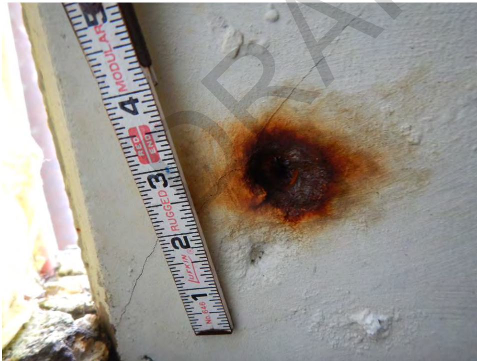
Figure 6-7: Typical random area of corrosion on underside of Beam Slab panels
