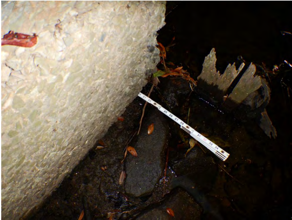
Figure 10-4: Undermining at northwest wingwall three (3) inches in height with up to two (2) feet of penetration
