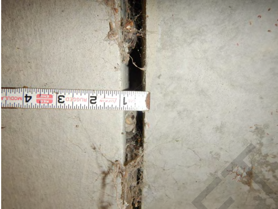
Figure 9-4: Opening between culvert segments
