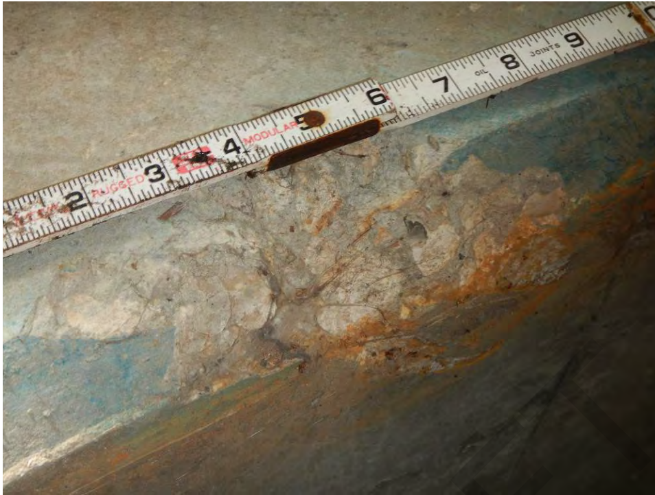
Figure 10-6: Concrete edge spall underside of arch
