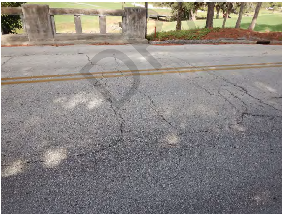
Figure 10-3: Transverse cracks in bridge deck
