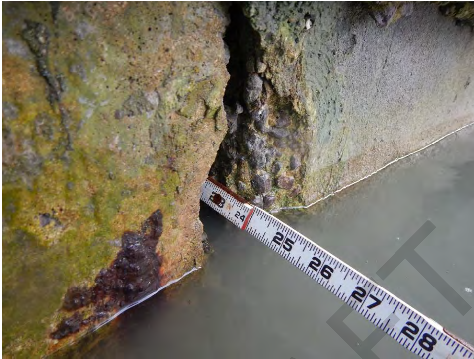
Figure 5-2: Void behind seawall at wall joint
