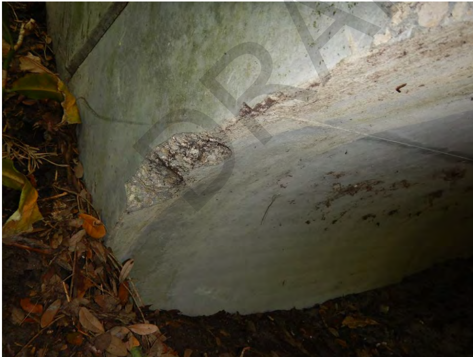
Figure 9-5: Construction spalling along ceiling edge of culvert opening
