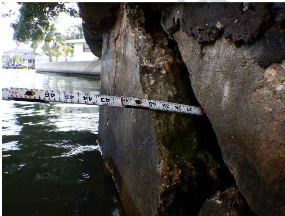
Figure 4-3: Southwest Wall – 4 inches of movement and 36 inch deep void
