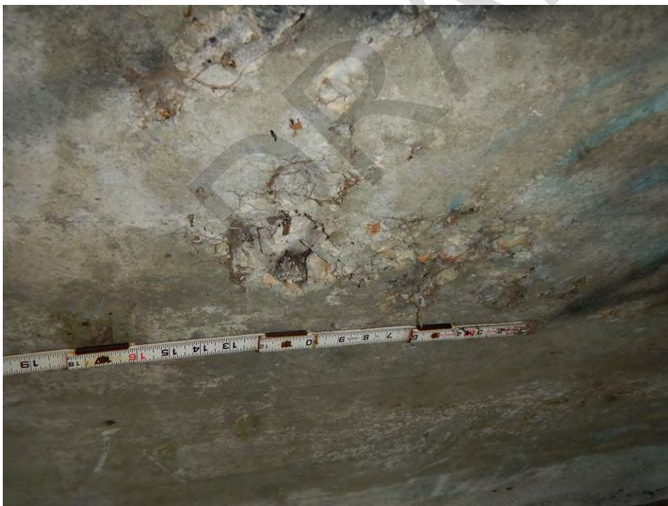
Figure 10-5: Honeycombing under arch near the mudline
