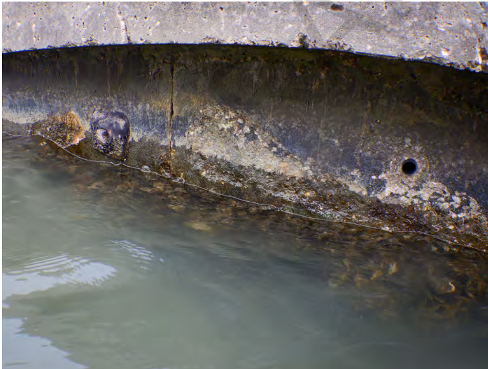
Figure 7-9: Example area of abrasion along seawall in splash zone
