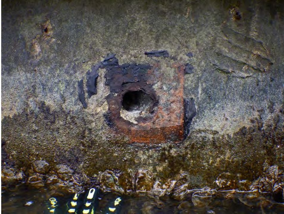
Figure 7-4: Missing tieback hardware
