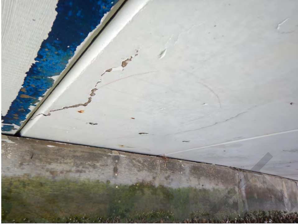
Figure 6-10: Area of delamination on underside of bridge deck.
