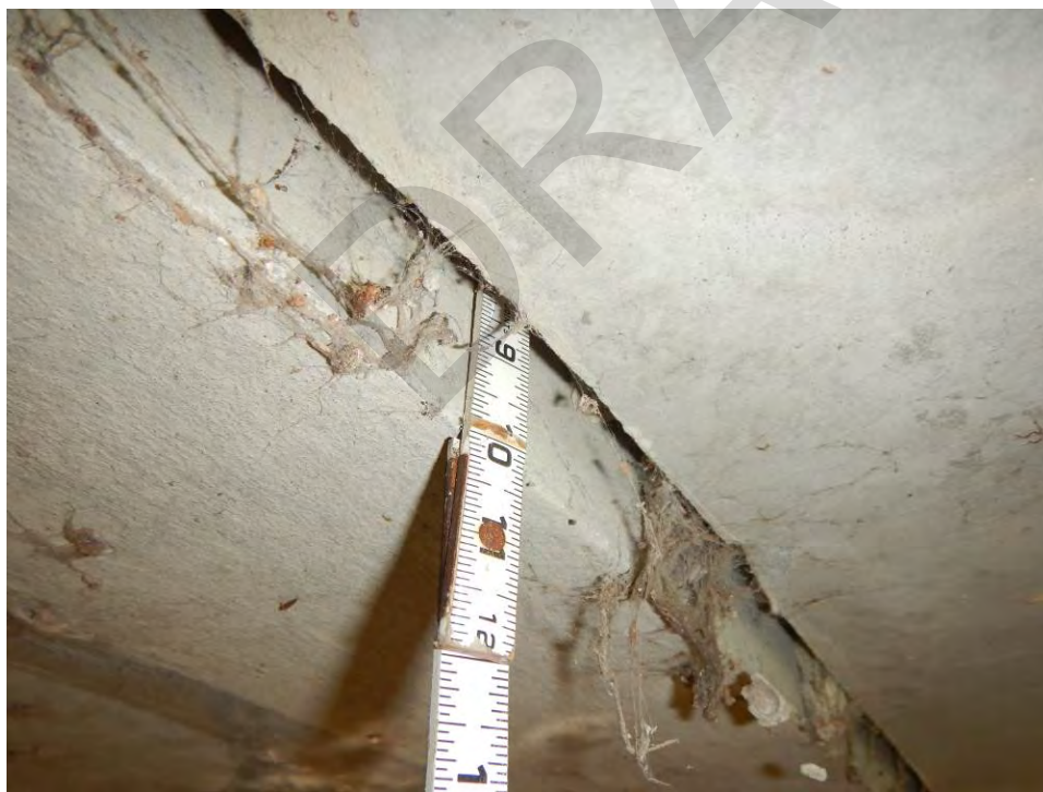
Figure 9-3: Misalignment between culvert segments with up to ten (10) inches of penetration
