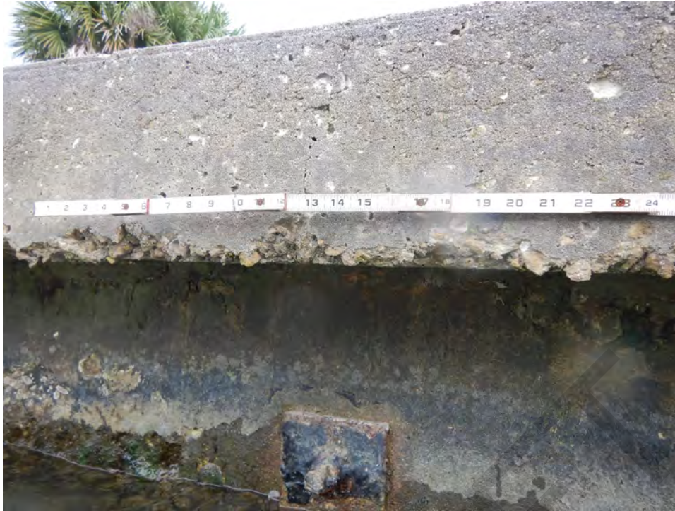
Figure 7-10: Typical spalling and cracking of cap underside
