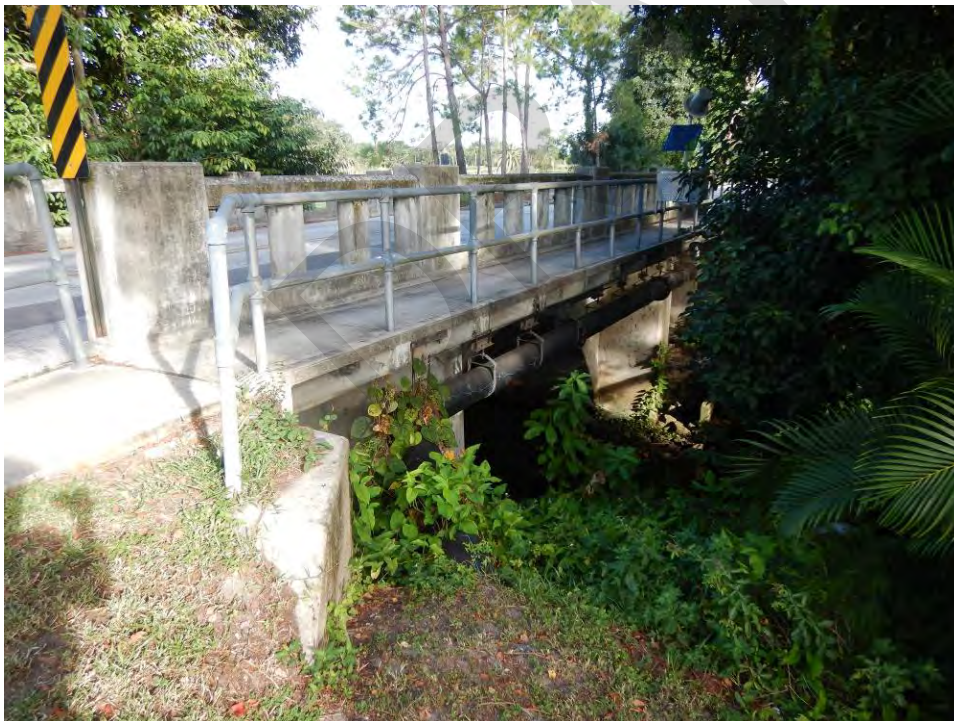
Figure 10-7: Bridge Section with obsolete crash barrier and sidewalk rail
