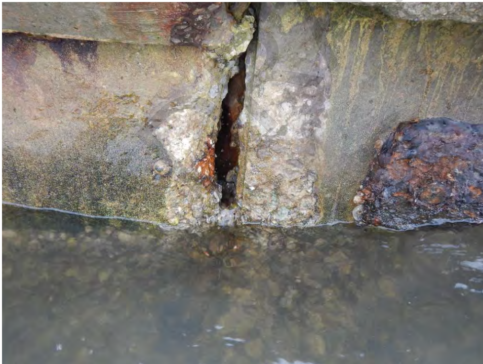
Figure 7-7: Typical spalling at concrete seawall panel joints
