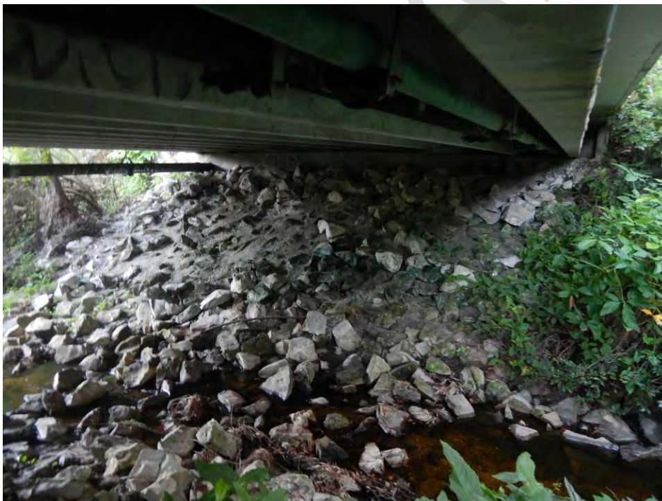
Figure 8-5: Channel and concrete rubble embankments
