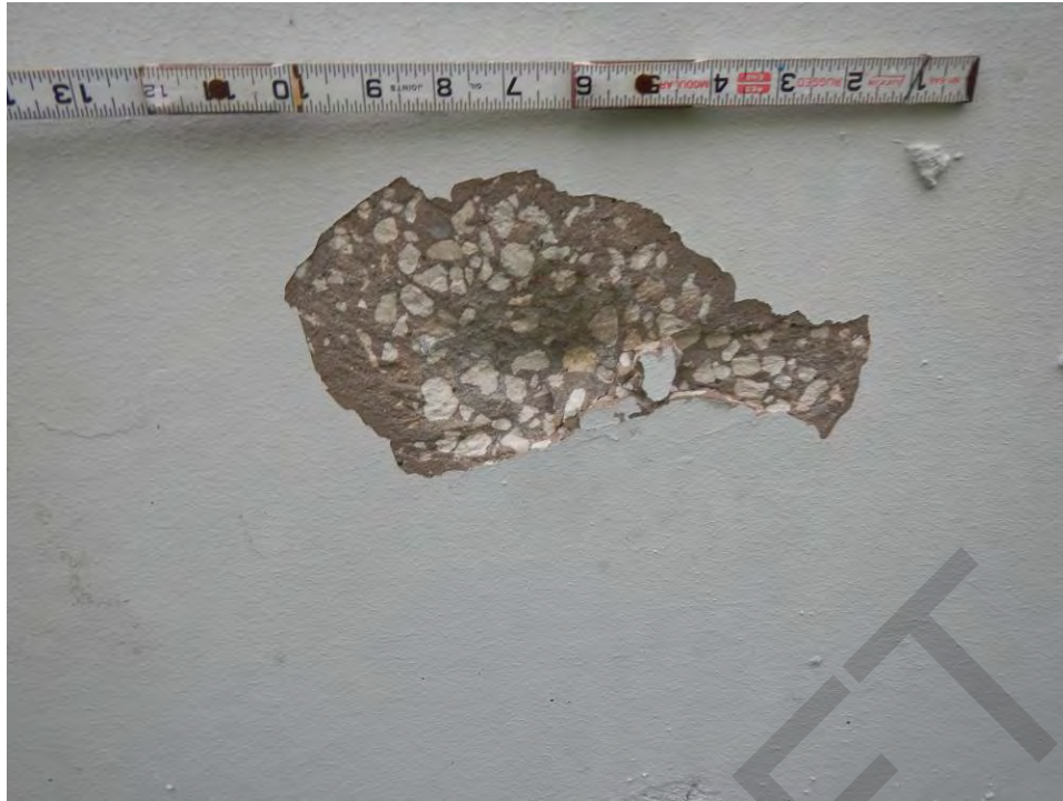
Figure 6-8: Typical spall in underside of Beam Slab panels
