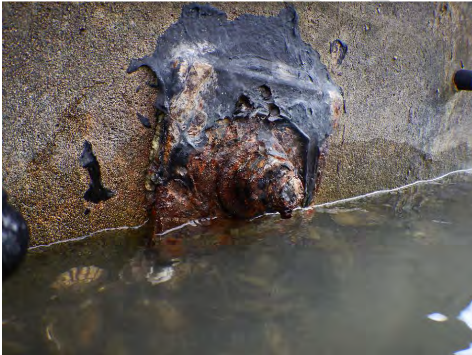
Figure 7-5: Typical tieback hardware, heavily corroded
