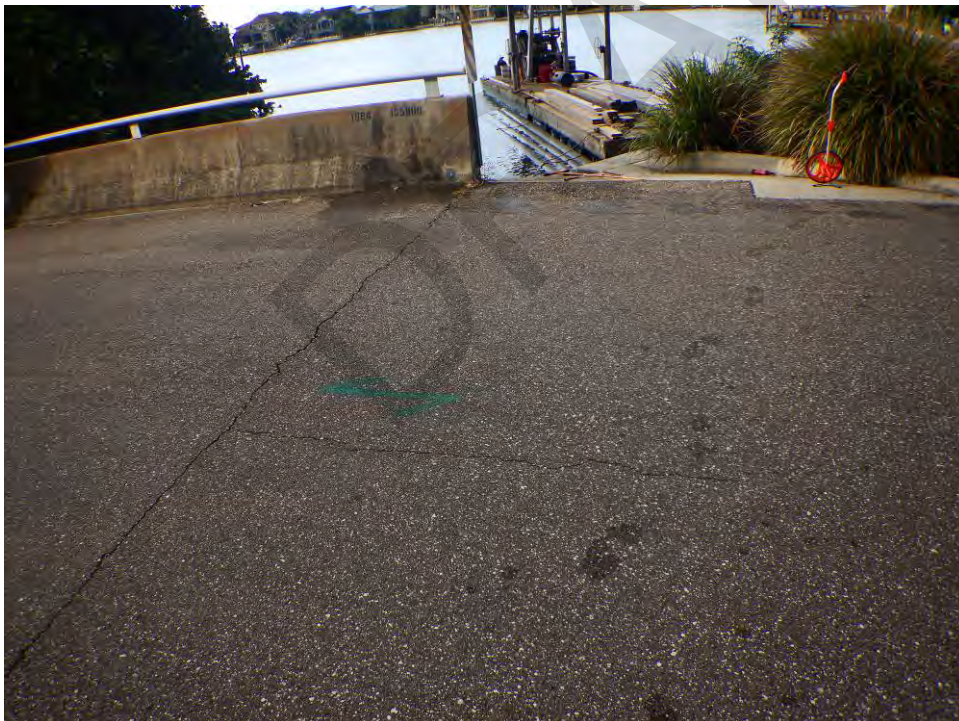
Figure 4-7: Cracks along expansion joint where the approach slab meets the bridge
