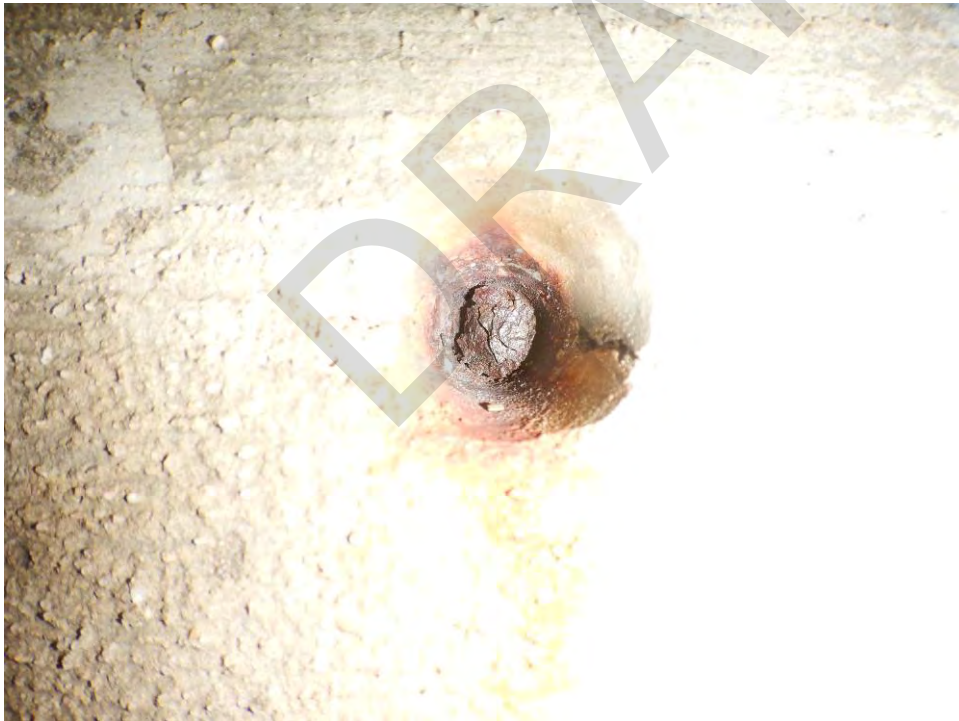
Figure 4-5: Corrosion to steel at unpatched form tie holes in face of abutment
