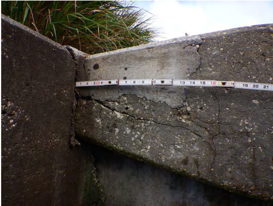
Figure 4-8: Cracks in wingwalls
