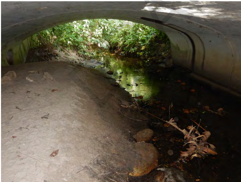
Figure 9-7: Aggradation within culvert
