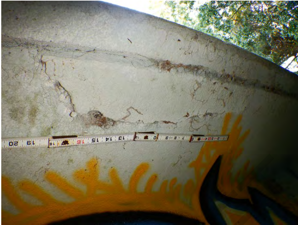
Figure 8-4: Area of delamination in beam
