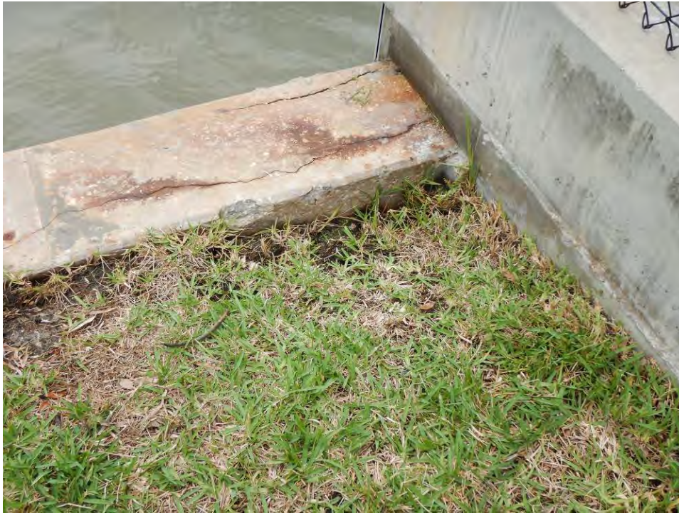
Figure 7-6 Evidence of fill loss behind seawall cap and longitudinal cracks with corrosion staining in top of concrete cap.
