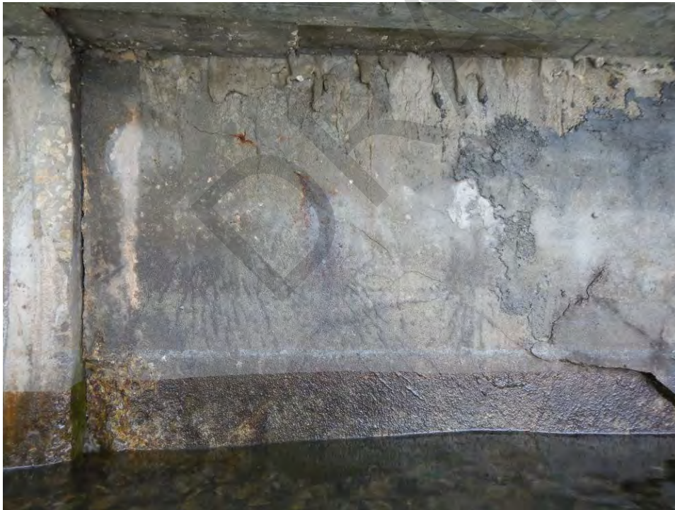
Figure 4-9: Diagonal crack with corrosion staining at the first joint from the bridge on the southeast corner where the wingwall meets the seawall.
