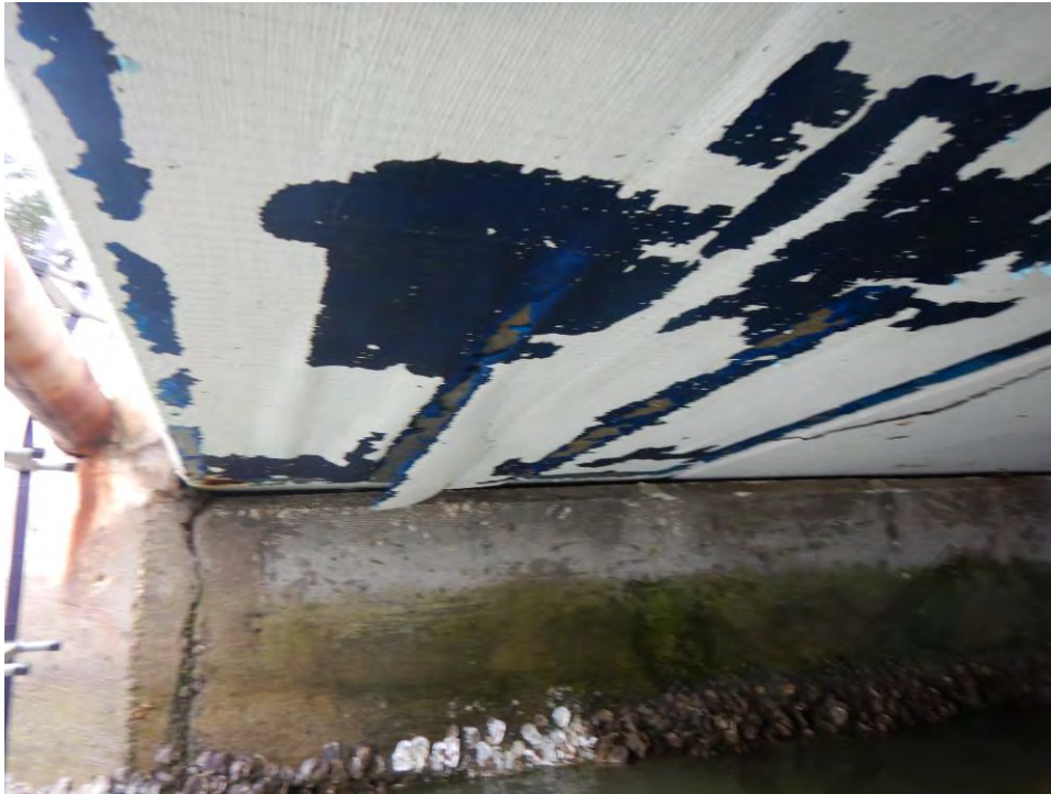
Figure 6-6: Under side coating failure
