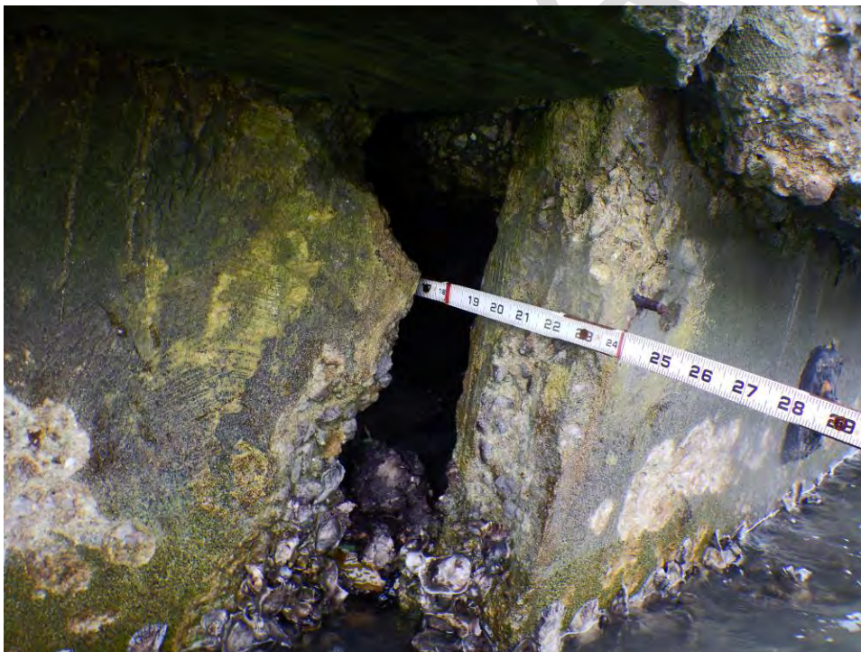
Figure 7-3 Deep void and loss of fill at wall failure
