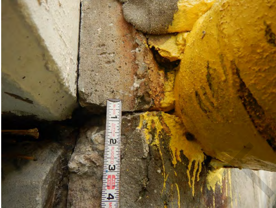
Figure 6-4: Cracks in the southeast wingwall due corroded utility
