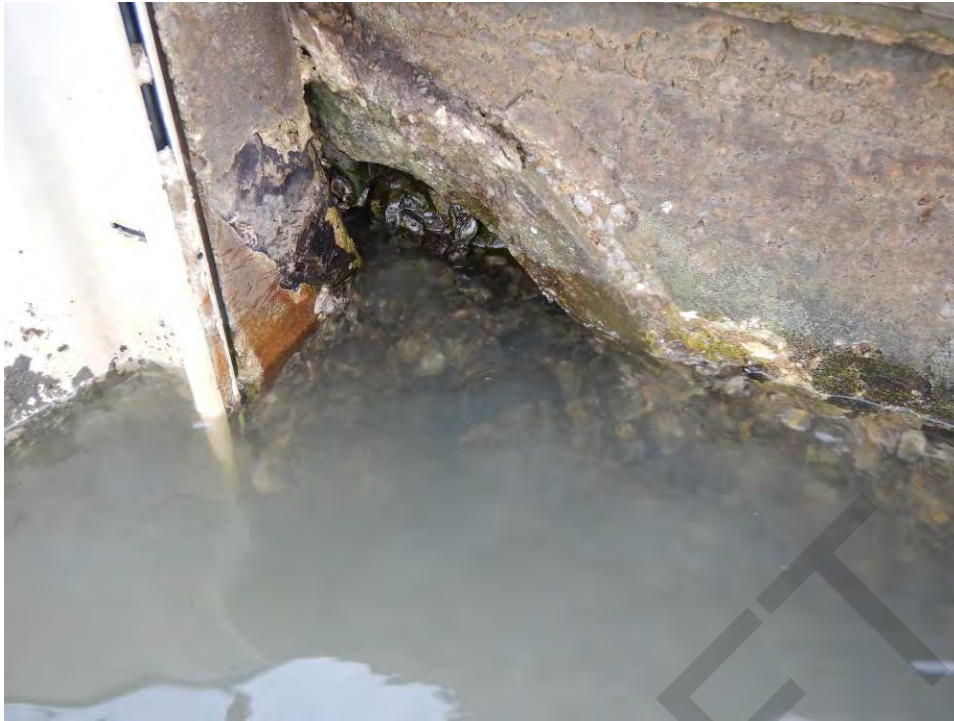
Figure 7-8: Partially covered outfall at the private property line north of the park
