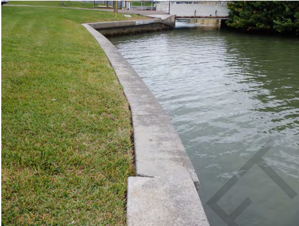
Figure 7-2 Wall failure resulting in large deflection between wall panels
