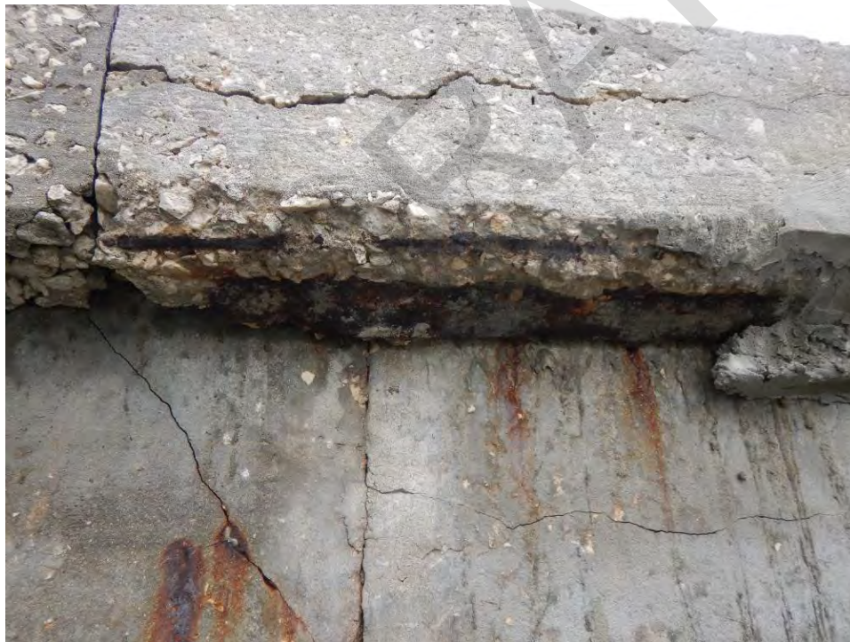
Figure 6-9: Cracks in wingwall / concrete panel wall connection on the southeast side of bridge. There is failure of the cap here with exposed steel reinforcing.
