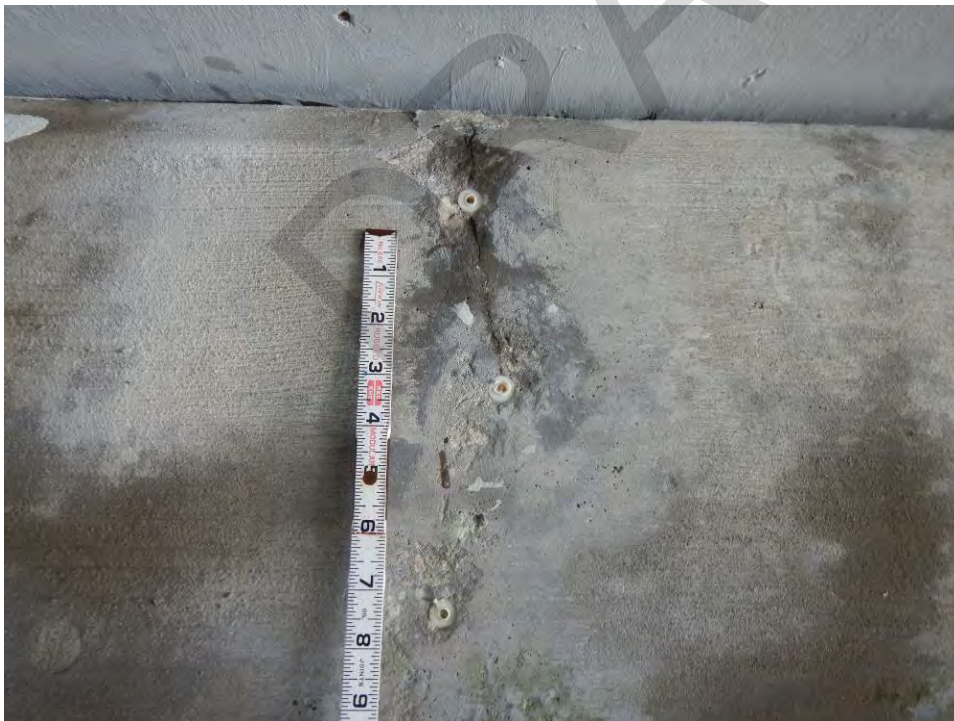
Figure 6-3: Cracks in abutments with epoxy injection repair
