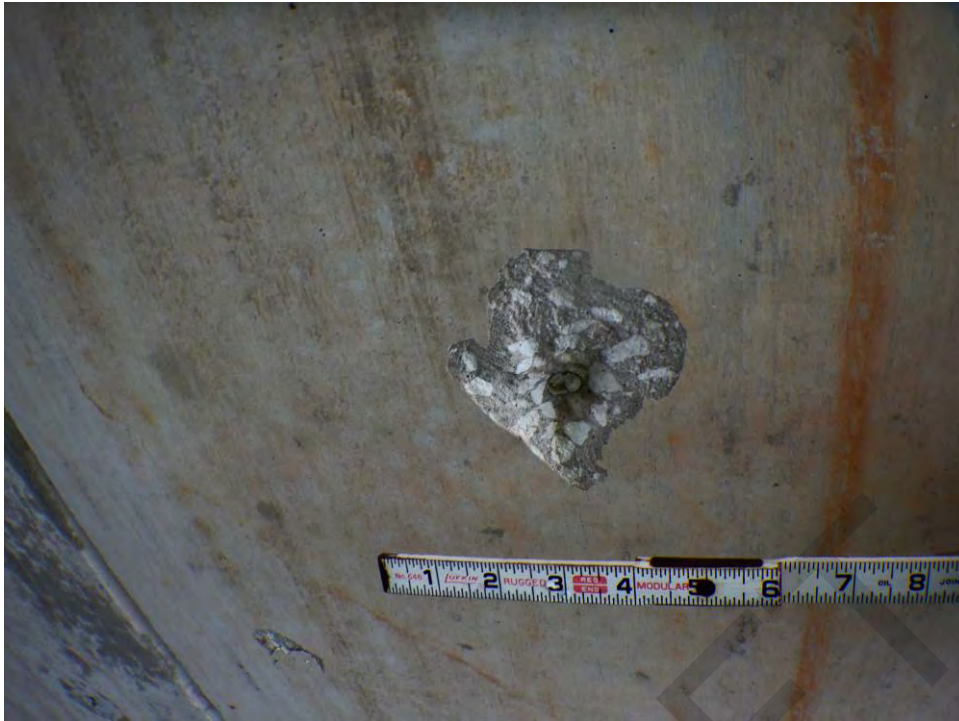
Figure 4-6: Typical spall at the underside of bridge slab beams
