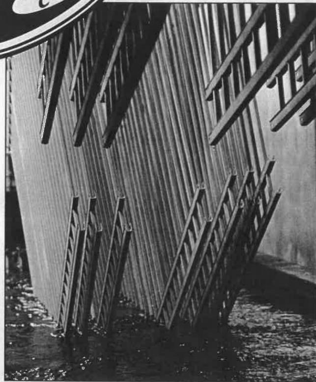
Conventional steel fences generally receive little or no cleaning prior to coating; they are typically painted by spraying the easily accessible outer surfaces, leaving ends and undersides vulnerable to corrosive attack.
