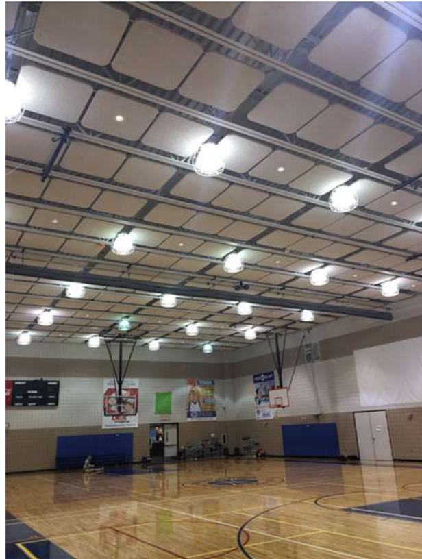
*Note: The metal halide (MH) lamps in the gyms are highly inefficient and have long “warm up” times that causes staff to turn them on well before the gyms are being used. The existing metal halide fixtures are also showing signs of “color shift” which is common as MH lamps degrade. The MH lamps have a short average rated life of 20,000 hrs. When these high reach lamps fail, the cost and labor time is high as town staff must secure a lift to replace lamps.*
