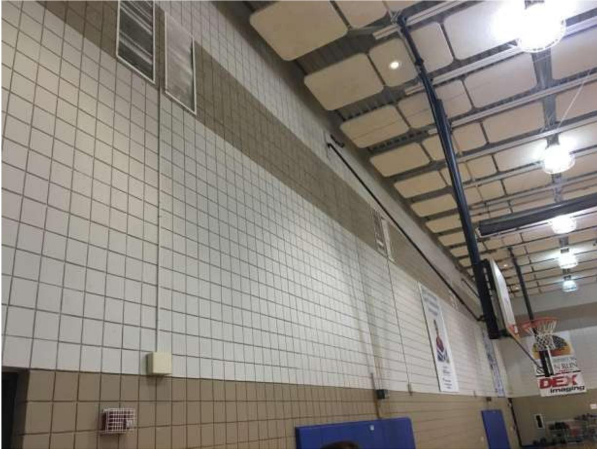
Gym units are being controlled by individual thermostats. Note the gym air grilles at the top of the photo. All of these grilles will be replaced with gym specific grilles.
