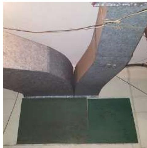
The hallway mechanical room is currently open outside air through a slotted vent. This uncontrolled outside air will introduce heat and humidity to the space even when outside air is not needed. The heat load will cause the air conditioning to run more than necessary, wasting electricity. The uncontrolled humidity source could also cause comfort issues.
