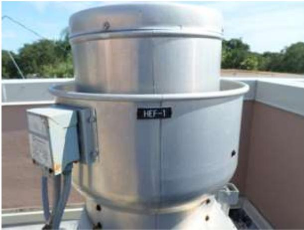
These are the two bathroom / locker room exhaust fans. They are in poor condition and will be replaced by higher efficiency exhaust fans.
