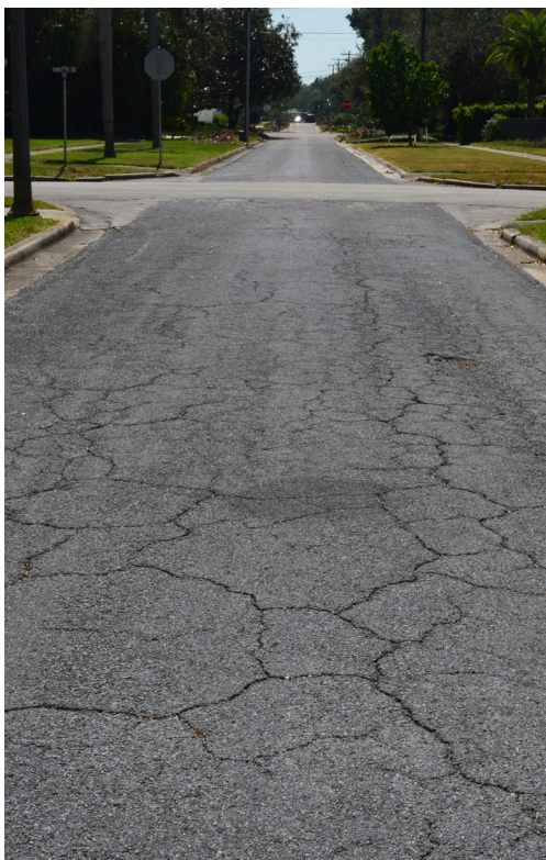
Alligator cracking along Pinellas
