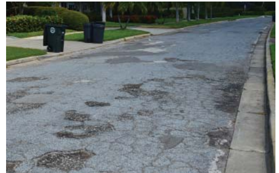
Asphalt degradation along Palmetto Road
