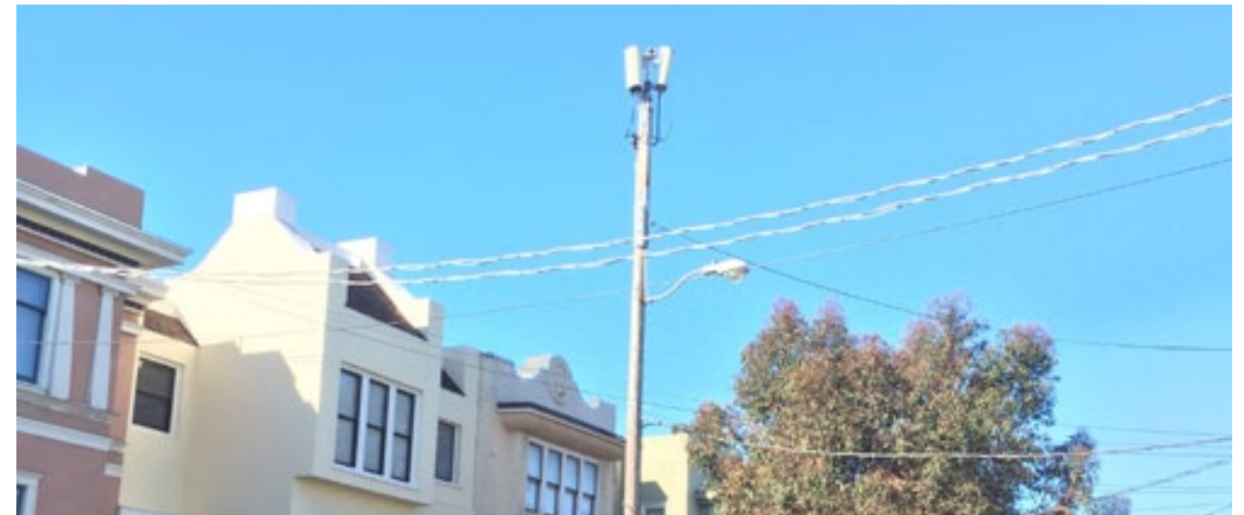
TOP: Disfavored use of multiple panel antennas with wide offset mechanical tilt brackets (evaluate electronic tilt alternatives) and loose cabling
