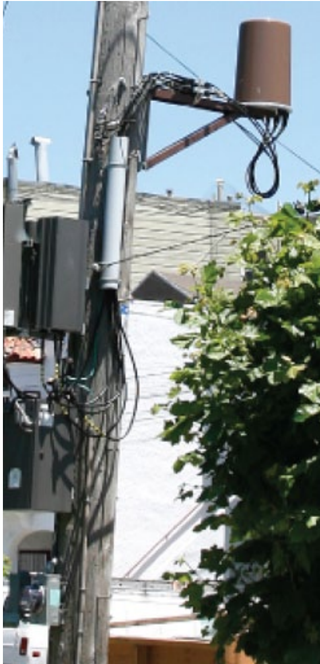
ABOVE: Disfavored excess loose cabling, excess decals/stickers, and cluttered appearance of equipment cabinets.
