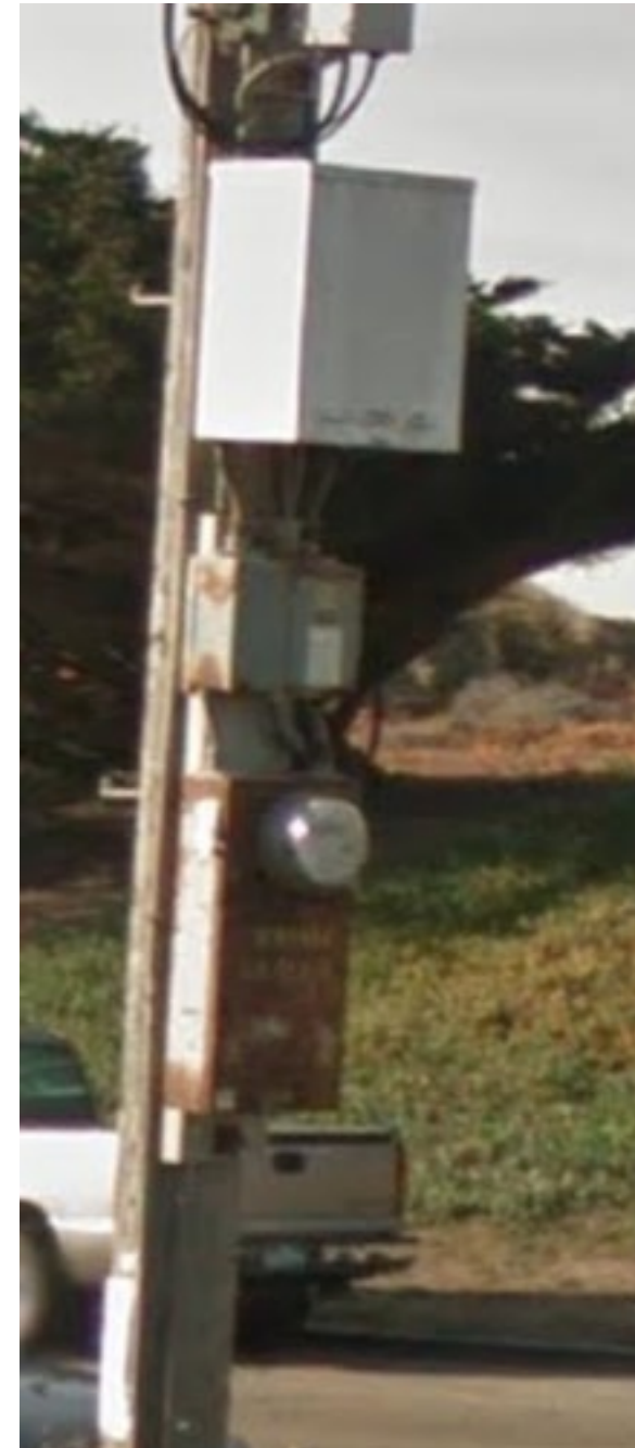
RIGHT: Disfavored facility featuring a leaning pole, rusted elements (equipment in photo has since been painted), very noticeable panel antennas (near cobra head street light), large node ID sticker on side of pole, and various form factors for equipment cabinets. In this example, the lowermost elements are the electric meter and disconnect switch. The square box is typically a battery backup unit used to provide limited backup power to the network, in case of a power outage. The skinny enclosure midway up the pole is essentially a computer used to route power and signal, via cables, up to the (disfavored) panel antennas.
