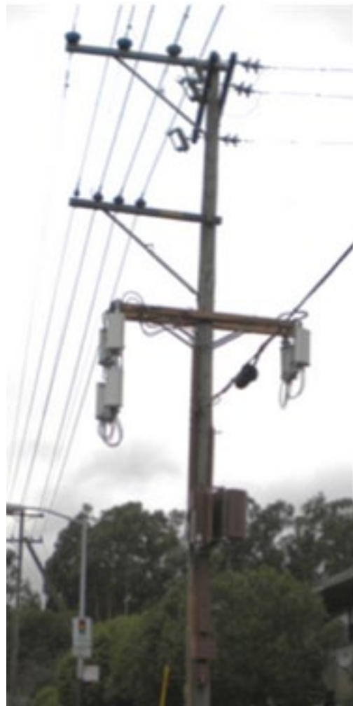
LEFT: Disfavored use of multiple panel antennas with cables loops dangling below each panel.
