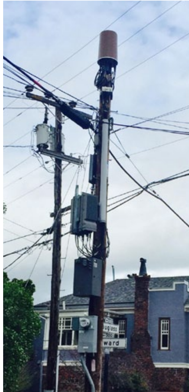
ABOVE: Disfavored example of cabling that is cluttered & tangled. Riser not painted.
