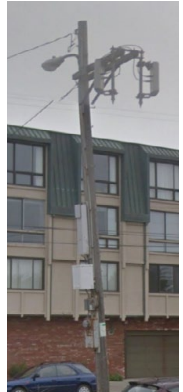
RIGHT: Disfavored facility featuring a leaning pole, rusted elements (equipment in photo has since been painted), very noticeable panel antennas (near cobra head street light), large node ID sticker on side of pole, and various form factors for equipment cabinets. In this example, the lowermost elements are the electric meter and disconnect switch. The square box is typically a battery backup unit used to provide limited backup power to the network, in case of a power outage. The skinny enclosure midway up the pole is essentially a computer used to route power and signal, via cables, up to the (disfavored) panel antennas.
