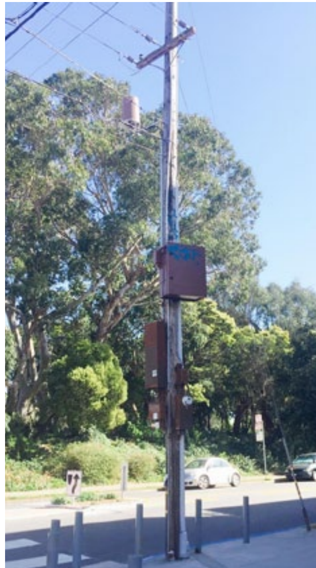
ABOVE: Disfavored use of a bulky/wide battery backup enclosure (with graffiti) and non-linear arrangement of other enclosures. Use slimmer/longer enclosures, including those specifically made for battery backup units (which are longer but about as wide as the pole), and possible re-location of portion of equipment (battery backup enclosure) to adjacent pole.
