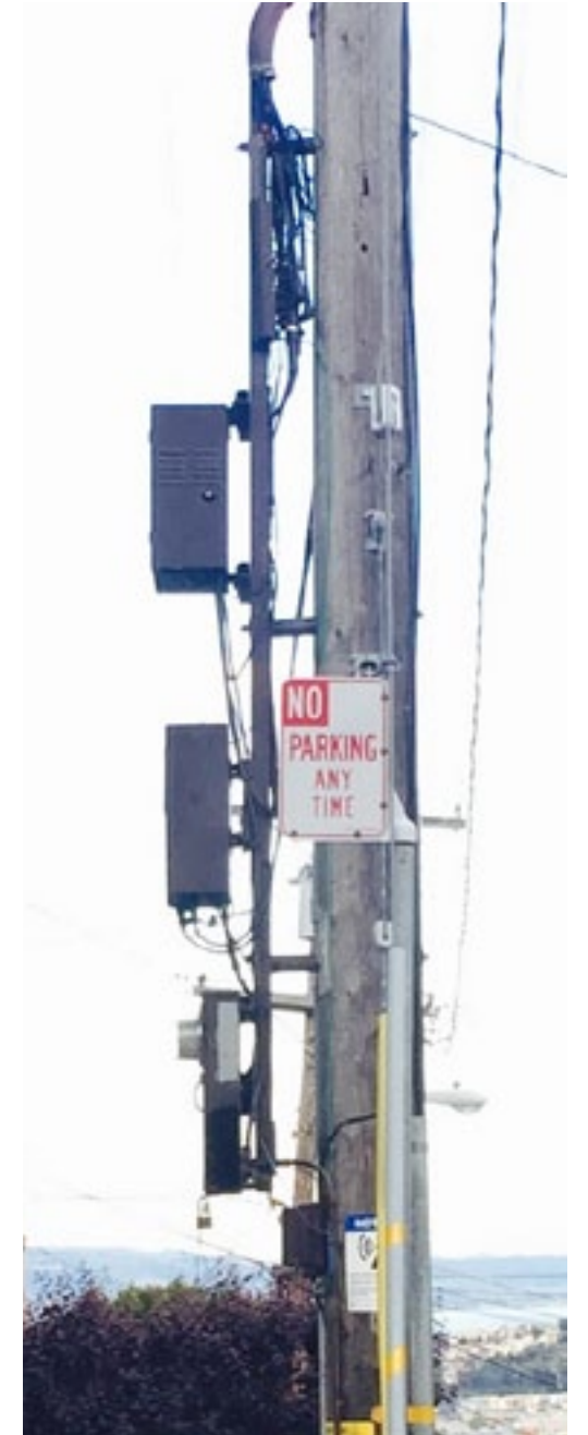
TOP RIGHT: Current Site Photo (after modifications) with disfavored elements such as a wide offset between the pole and equipment enclosures; excess cabling, large bright node identification (yellow placard) and RF warning sticker next to equipment (instead of up near antenna) at pedestrian level.
