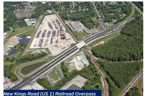
New Kings Road (US 1) Railroad Overpass
