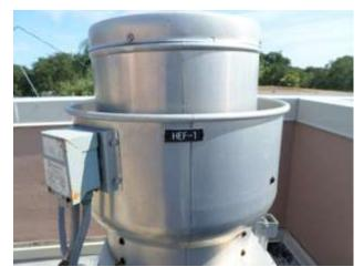
These are the two bathroom / locker room exhaust fans. They are in poor condition and will be replaced by higher efficiency exhaust fans.
