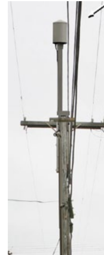
RIGHT: Preferred top-mounted antenna design with shroud cap below the actual antenna (below seam line); and without a significant pole height increase.
