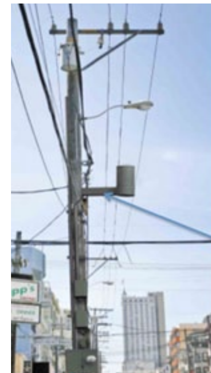
Antenna mounting arm with cabling and other electronic elements screened from view inside bracket
