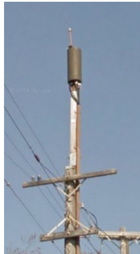
ABOVE: Non-recommended (triple panel) antenna design that is bulky/obtrusive, and rises well into view.
