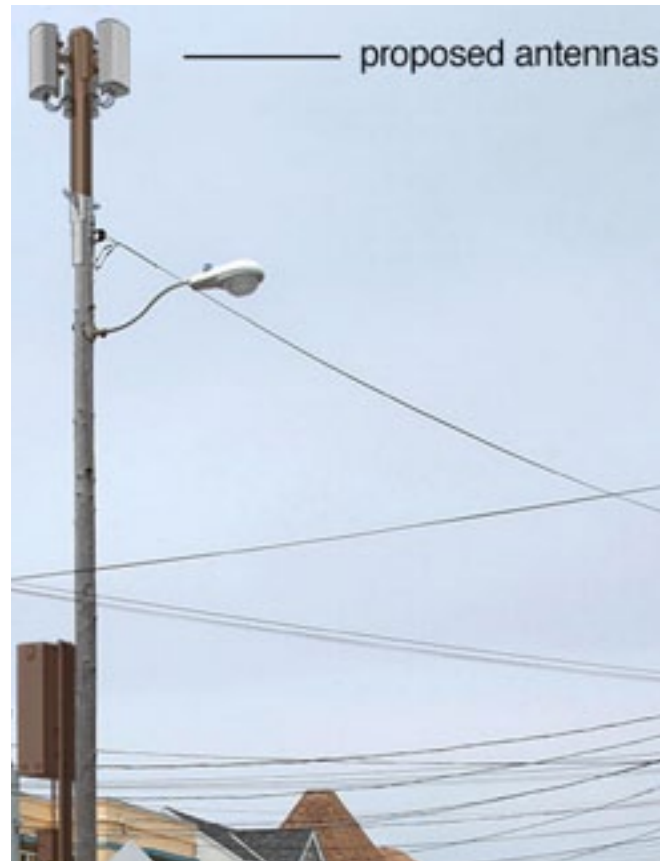
ABOVE: Non-recommended (triple panel) antenna design that is bulky/obtrusive, and rises well into view.
