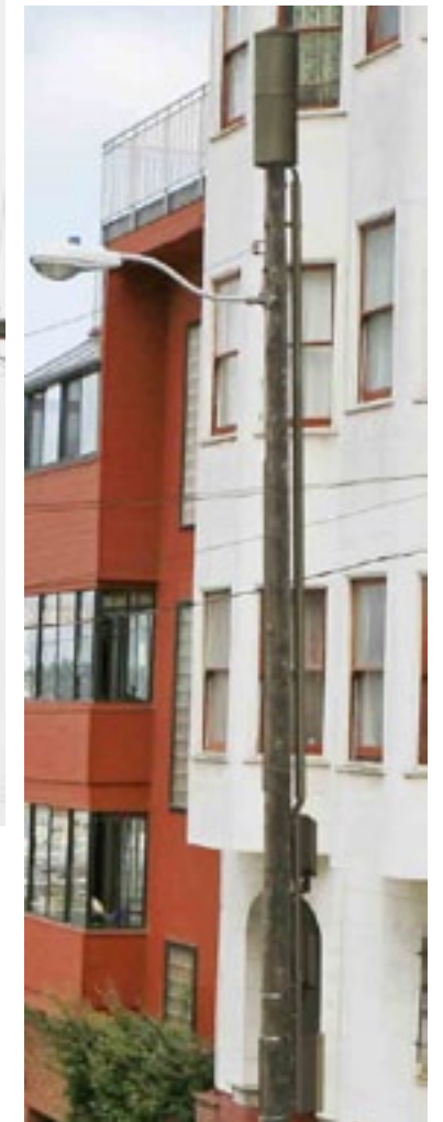
LEFT: Disfavored extension arm. Too narrow and noticeable due to shape change and height increase.
