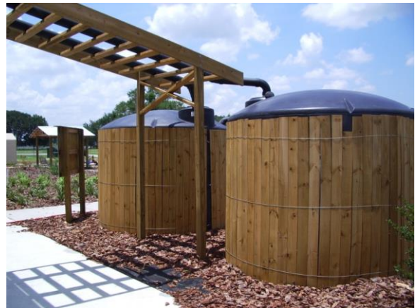
A rainwater harvesting cistern used for irrigation.
