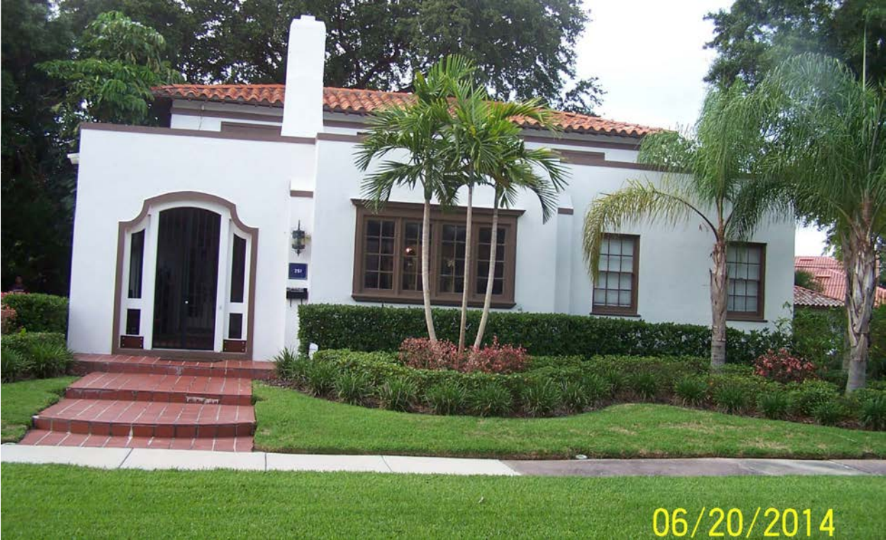
251 Pine Road before construction (November, 2014)
