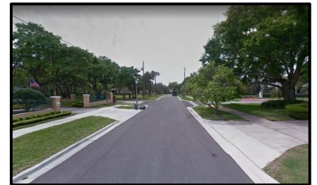
Peter Nikolov designed the Manatee Road Improvements for the Town of Belleair
