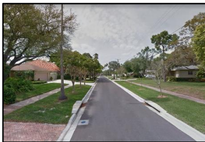
Osceola Road Improvements
